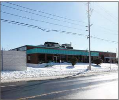
115-119 Skyway Ave, Etobicoke 17,500 SF Industrial Building, Receivership Sale
